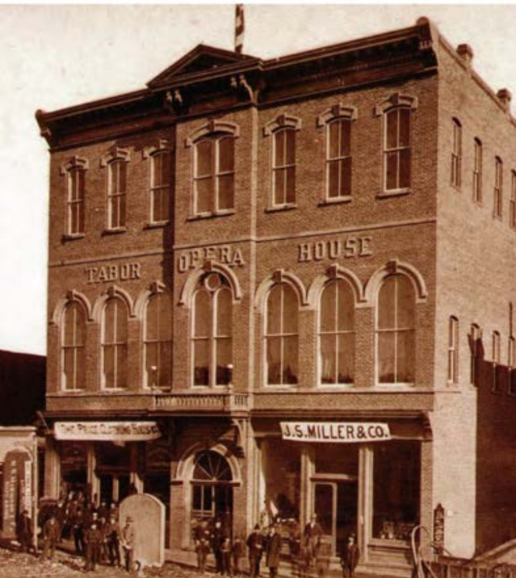
Historic Structure Assessment Tabor Opera House Leadville, Colorado
