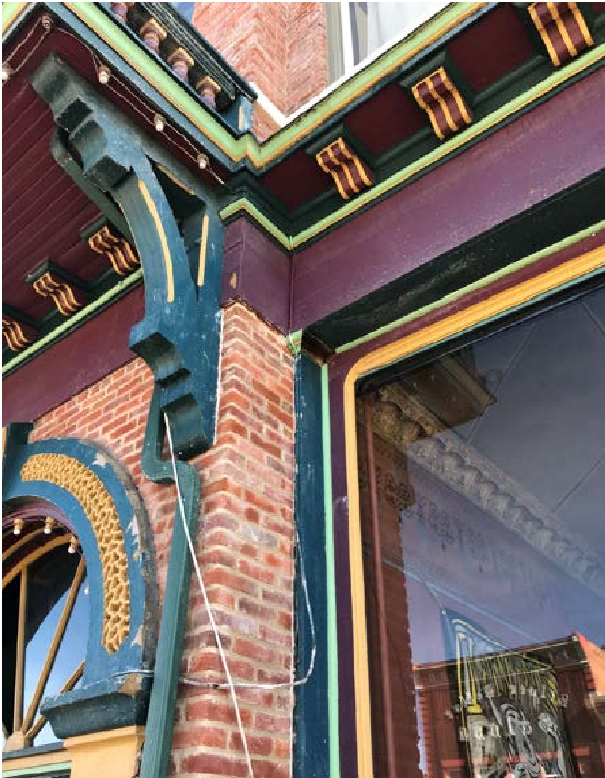
Image 10 – South side of Central Main Entry. Wiring serving the decorative lighting at the fanlight window is loose, susceptible to damage, and posing a safety hazard. The wiring will be replaced with concealed wiring, where possible. The downspout and supporting wood blocking will be removed following the rehabilitation of the balcony where a scupper for drainage is planned. A masonry allowance is provided with this project for repairing damaged brick behind the blocking. The brackets supporting the decorative cornice and the underside of the balcony can be seen in this view.
