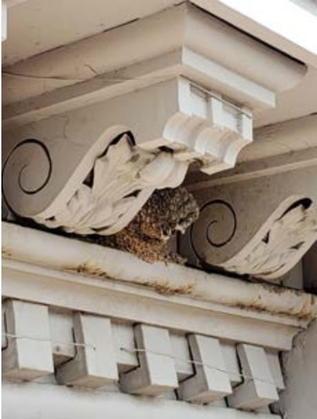
Baling wire repairs
