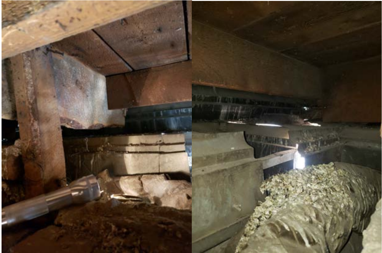
Upper cornice framing details
