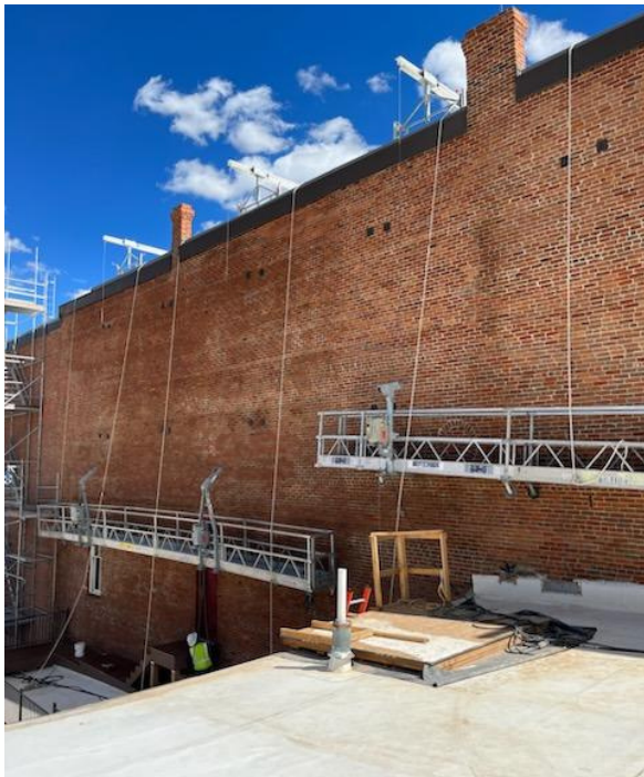
The scaffolding on the Tabor's north wall-used a swing stage system for 2023 construction
