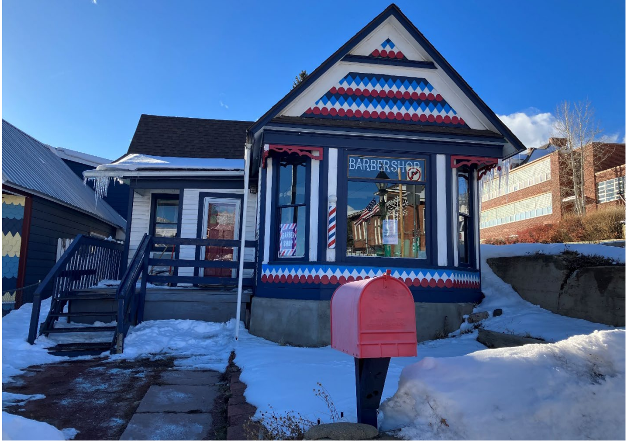
Image 3 (Above): Looking west at the property from Harrison Ave.
