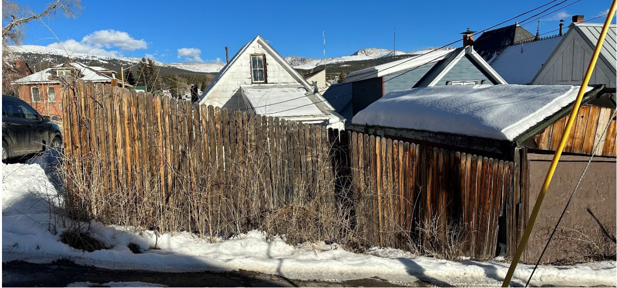
Image 5 (Above): Looking east at the property from the rear public alley.
