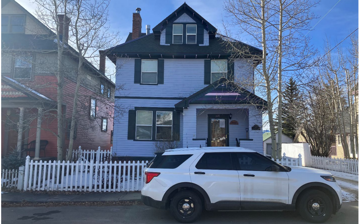
Image 3 (Above): Looking west at the subject property from Spruce St.
