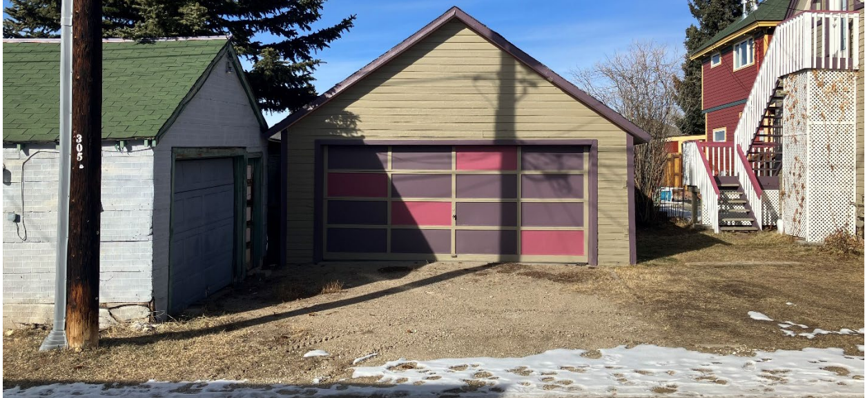
Image 7 (Above): Looking north towards the detached garage from the public alley.
