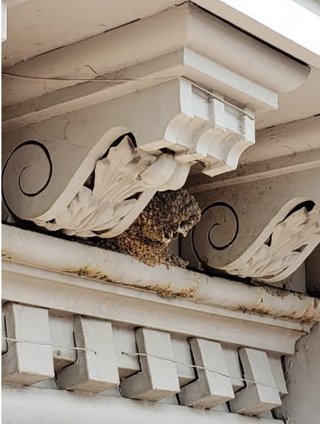
Baling wire repairs
