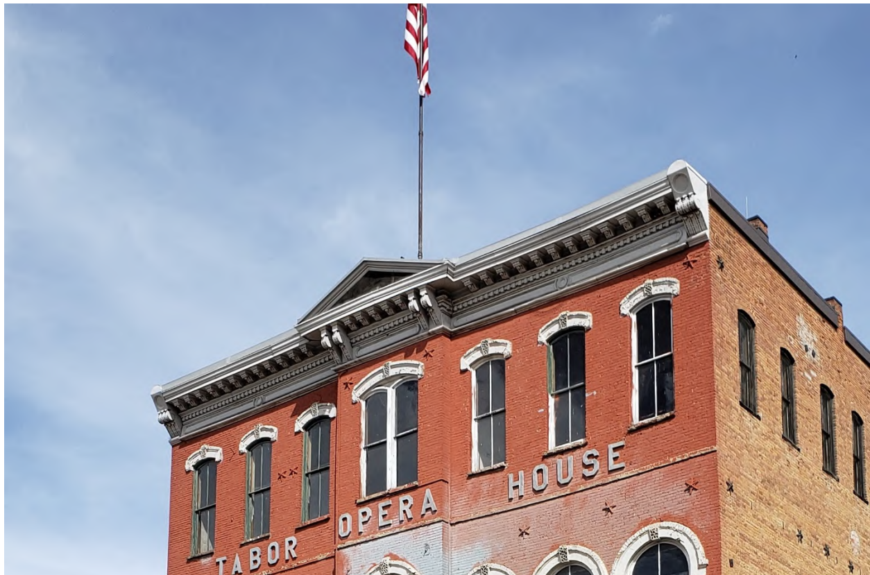
The Tabor Opera House, west elevation
