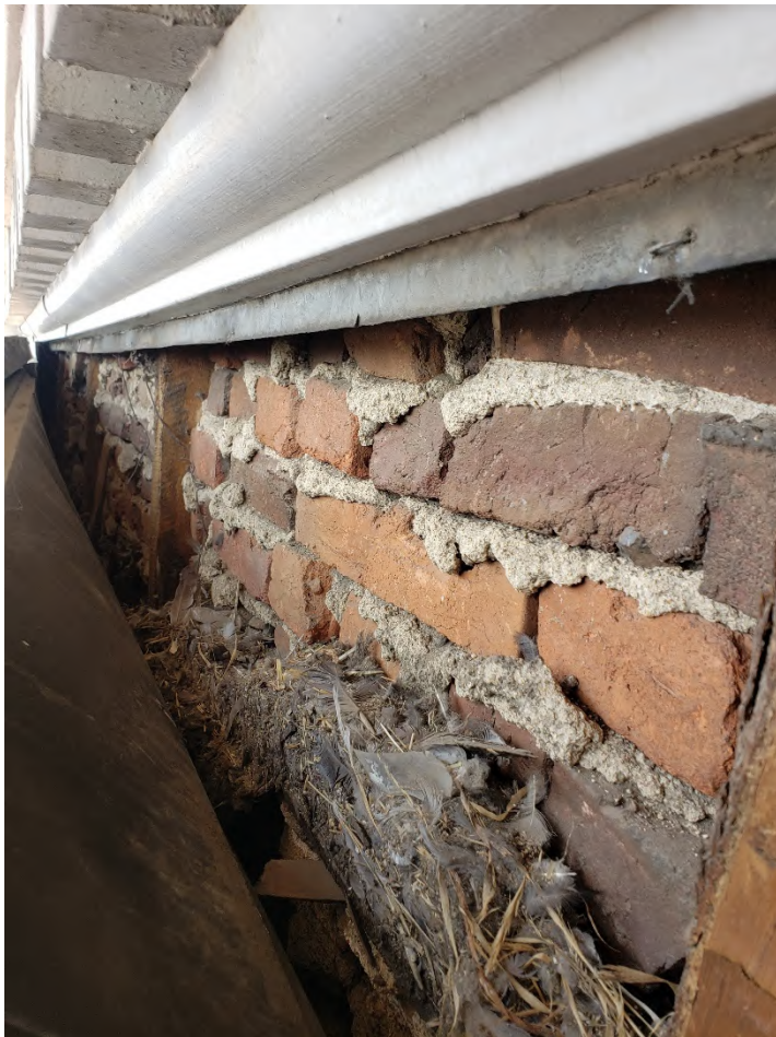
Lower cornice framing, with vertical 2x4's let into brick wall
