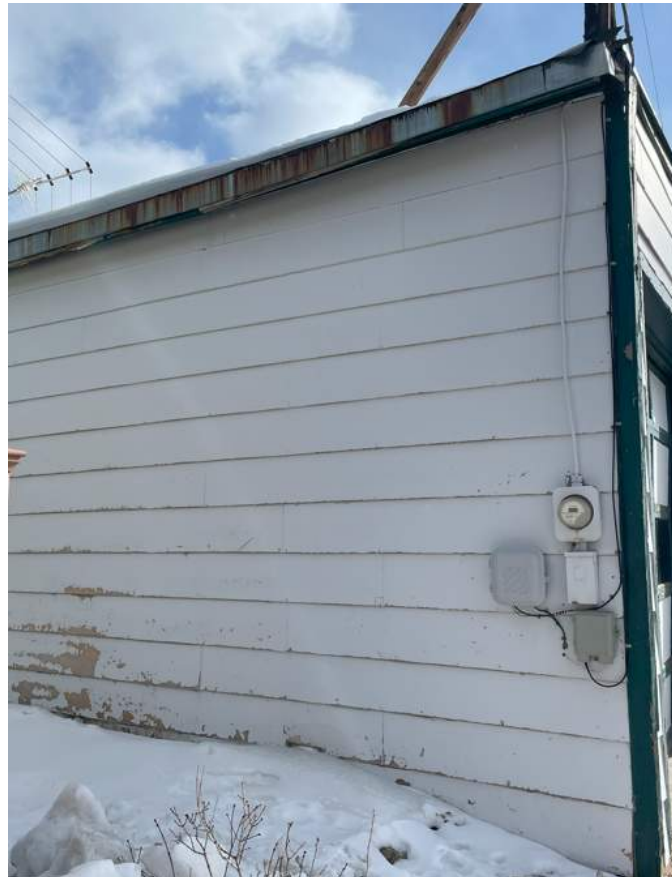
Exterior View from the north alley
