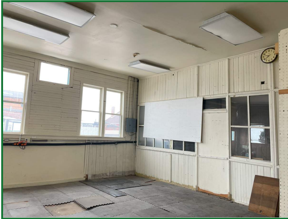
Existing Interior Condition
