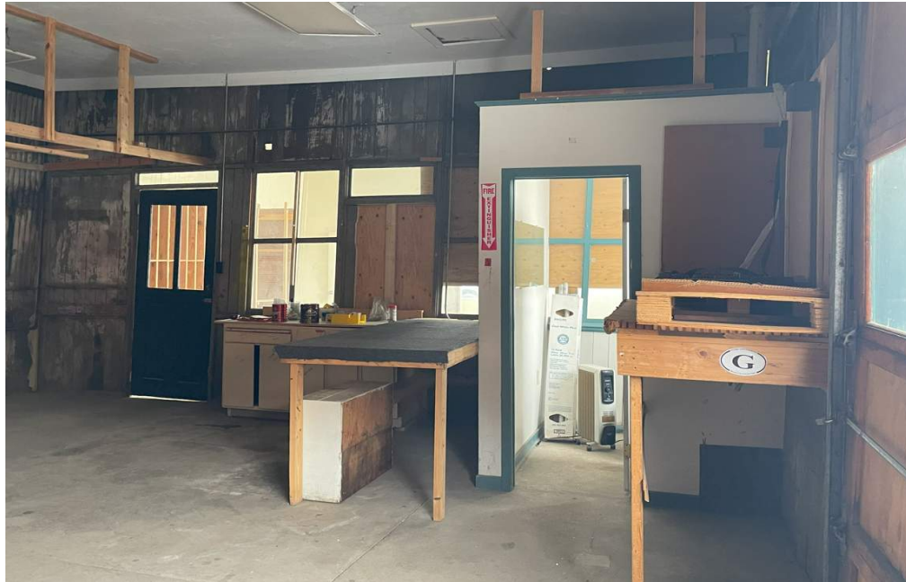
Existing Interior Condition
