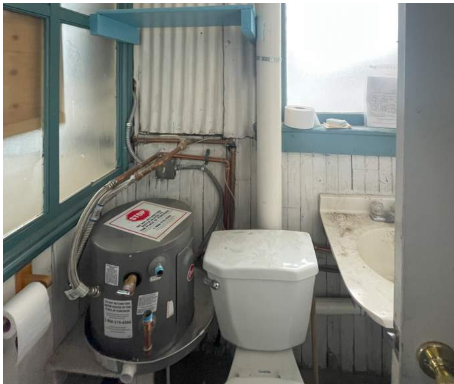
Existing Interior Condition
