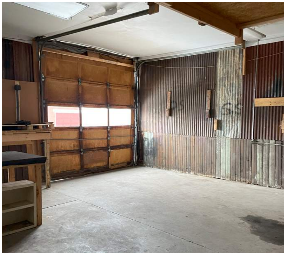
Existing Interior Condition
