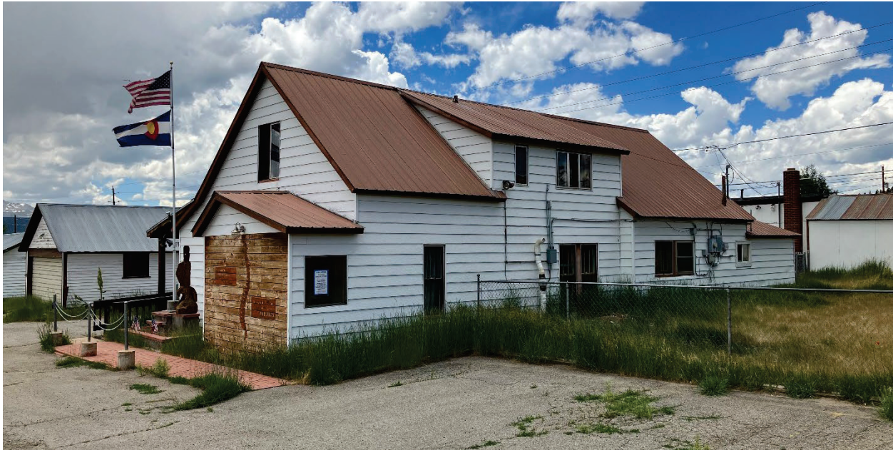
Image 4 (Below): Looking northwest at the property from Front St.
