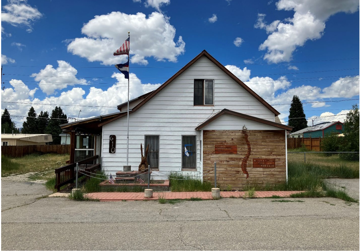
Image 3 (Above): Looking north at the property from Front St.
