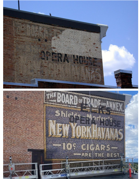
Before & After - North Wall Ghost Sign Restoration
