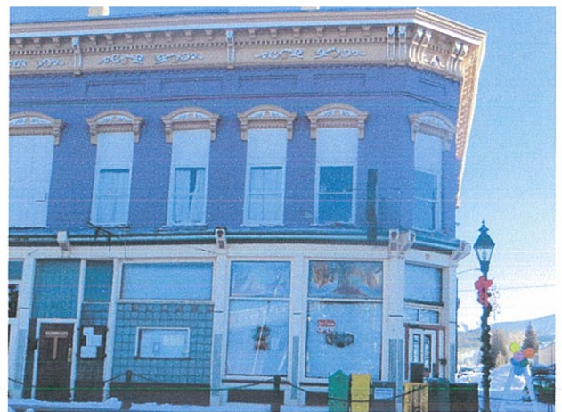
Ornamental cornice is representative of nineteenth century architecture.
