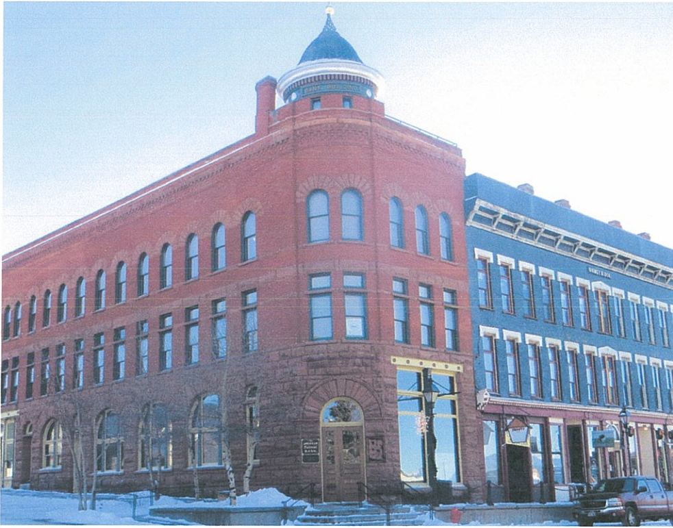
This three story American National Bank Building, made of brick and sandstone, was build in 1892 in a Romanesque style. This building has been completely renovated.
