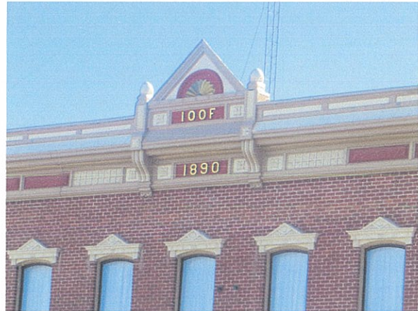
The cornice provides a strong termination of the facade.
