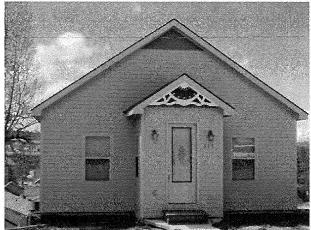
Figure 6. Building depicts sloping roof forms traditionally found in Leadville.
